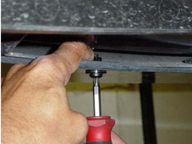
Photo 1-J: Mounting screw attached
